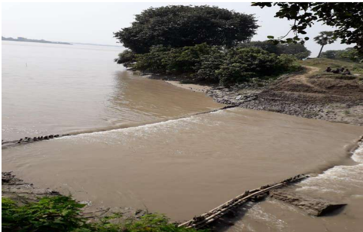
Silt Rich Water Entering Silt-Tanks
